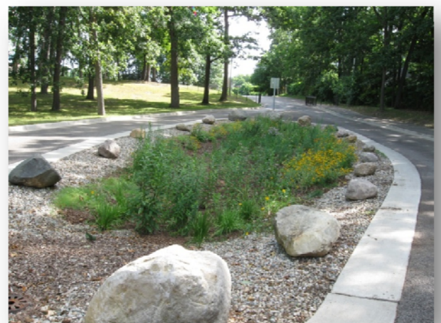
Figure 6: Example Rain Garden Installation
