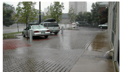
Figure 2: Example Urban Permeable Pavement Installation
