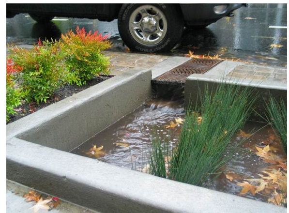
Figure 4: Example Curb Bump-out Rain Garden
