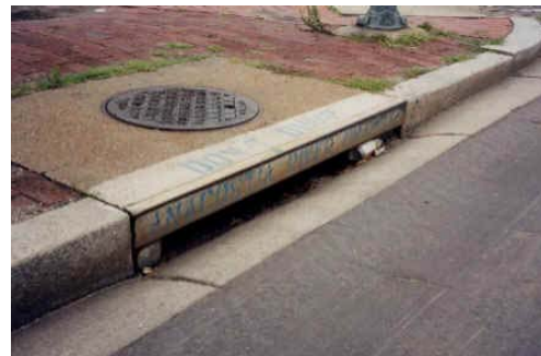
Typical Catch Basin, Clear of Debris and Trash
