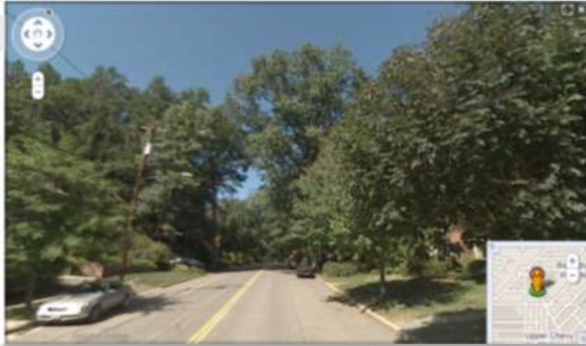
Exhibit 24 Heavily Treed Areas – Feeder 14133 near 2936 Brandywine St. NW
