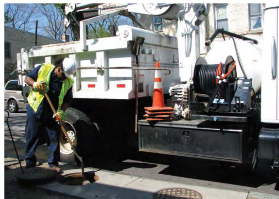
Crews remove debris from catch basins
