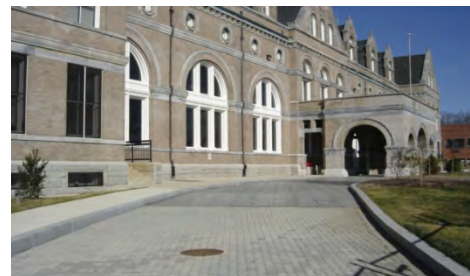
Permeable (or porous) paving allows rainwater to seep through the paved surface and into the soil below
