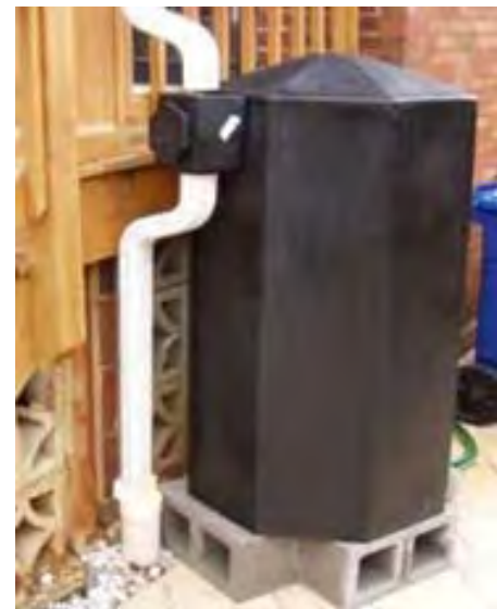
132-gallon cistern, with dimensions of 51" x 27"
