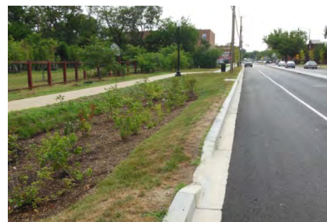
Along Nannie Helen Burroughs Corridor is a curb cut feature integrated with a bioswale
