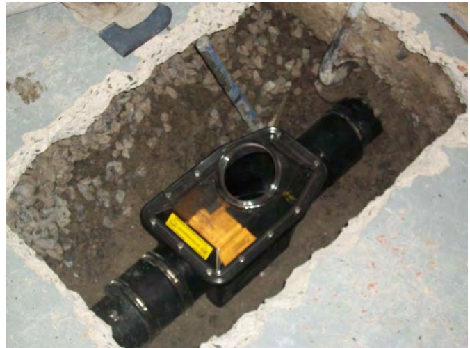
Figure 5-3: Installation of backwater valve into basement (Source: Multi-Drain, Inc.)
