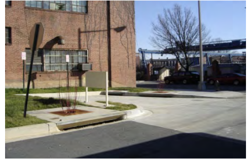
Tree filters located on DC Water's Bryant Street Pumping Station facility
